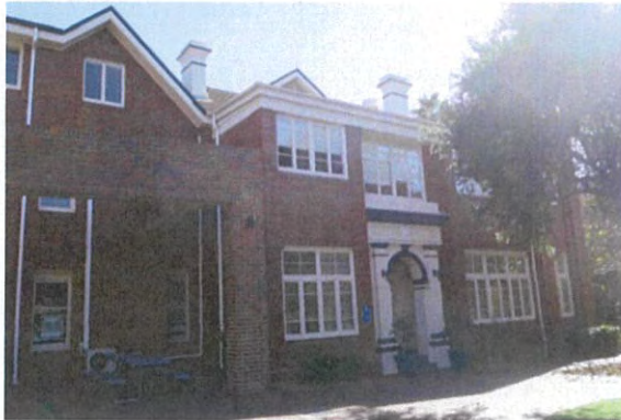
Figure 8 – Eastern elevation of Wallis Hall, 2018. Evidence of the former Victorian villa in roof form and plaster portico.
