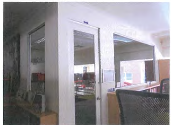
Figure 13 – View of Hudson Library looking north west showing recent refurbishment and fabric
