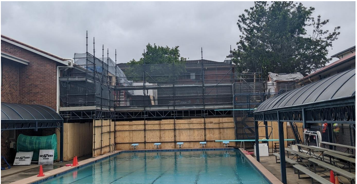
Figure 4 – DaCA building following completion of removal of make safe works, with hoarding and scaffolding erected.
