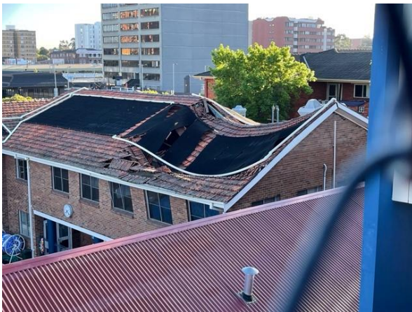
Figure 2 – Roof of DaCA building following collapse in December 2021
