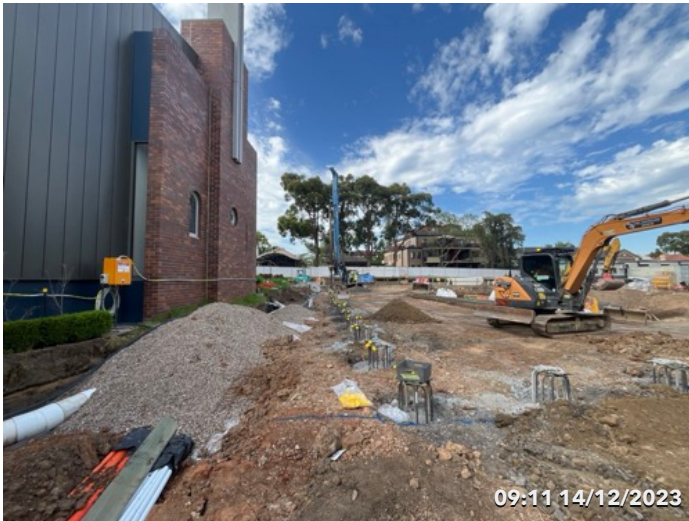
Photo 1 Piling works commenced.
