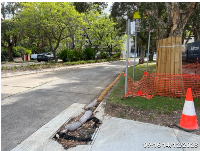
Photo 6 Coir logs were installed along the gutter and pit was covered with geofabric.
