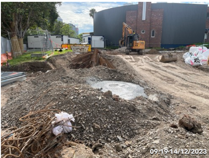
Photo 15 Concrete wash bay area.
