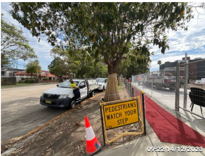
Photo 17 Designated work zone area and pedestrian signage and pathway was installed.
