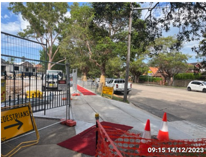
Photo 5 Site access/egress - free of dust or mud. Traffic controls in place specifically pedestrian signage and footpath.
