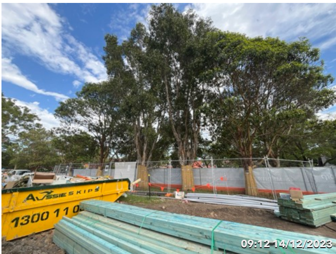
Photo 3 Tree protection installed as per Council requirements.
