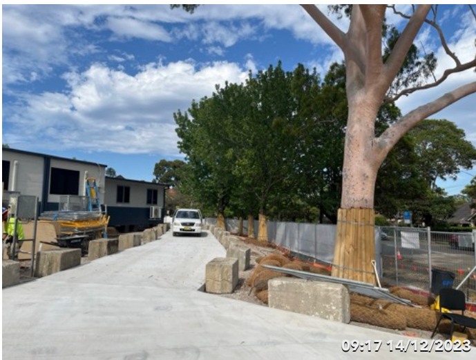
Photo 12 Tree protection and barriers were installed.
