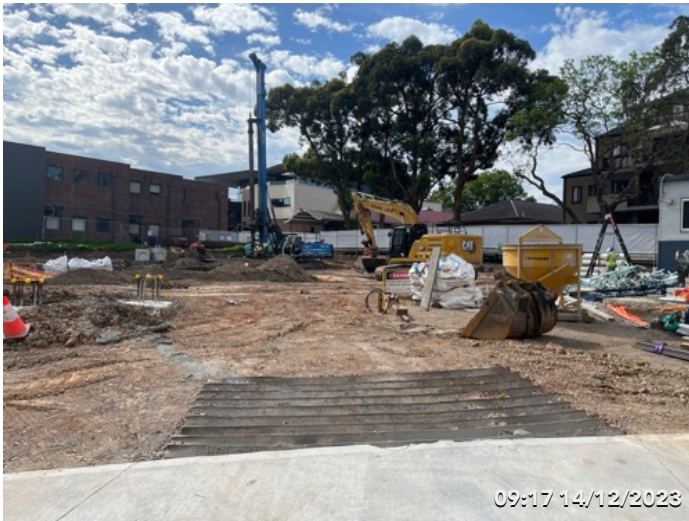
Photo 10 Rumble grid installed.
