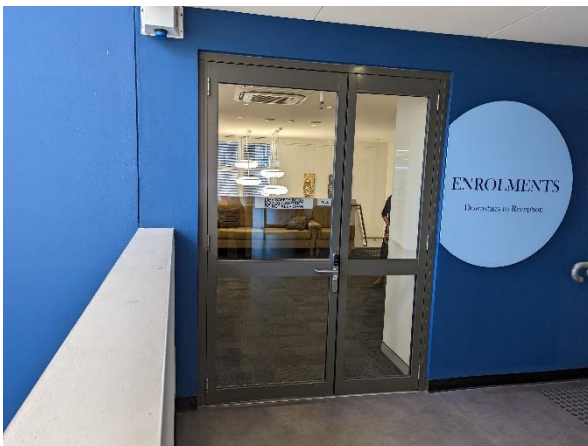
Figure 4 – Door C, Administration Building, Upper Ground Floor Source: Meriden School, 2022
