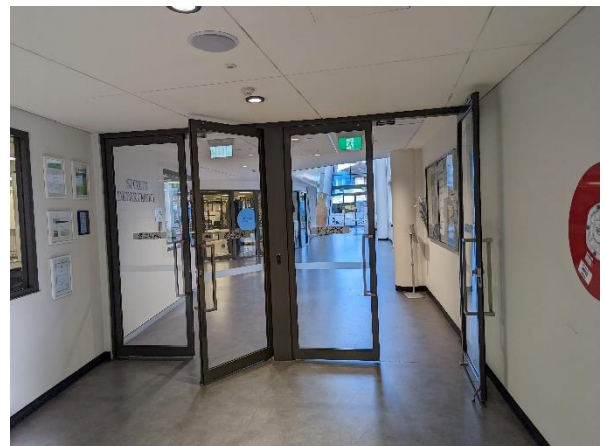
Figure 5 – Door D, Sports Centre Ground Floor Source: Meriden School, 2022
