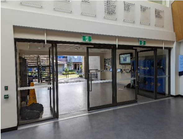
Figure 6 – Door E, Sports Centre, Upper Ground Floor
